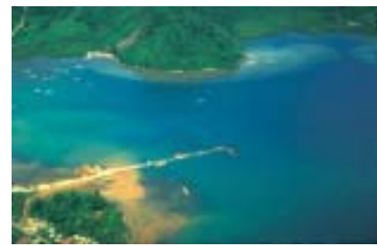
Bungus Bay, 20 km south of Padang (West Sumatra). Construction of an oil pier in the middle of a coral reef ecosystem.
